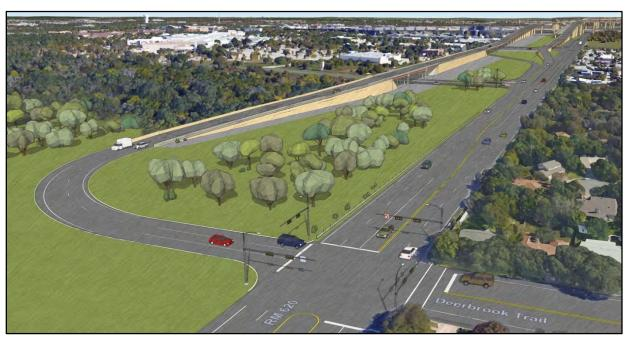
Figure 8. Build Alternative: Artist rendering (birds-eye view) of new button-hook exit from northbound US 183 direct connector ramp to RM 620 west.
